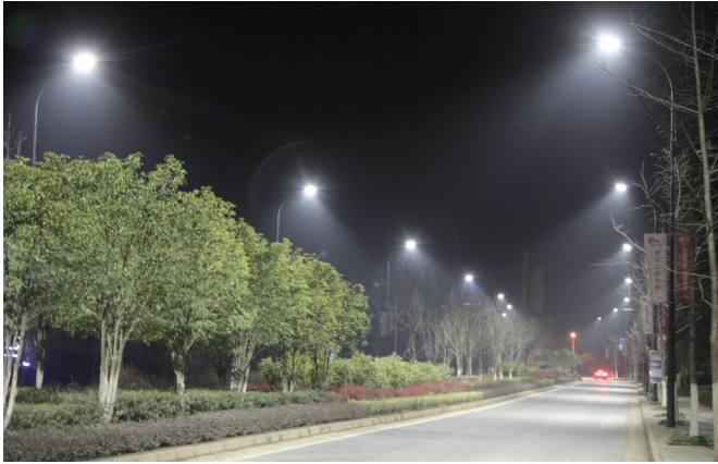
- for Road, China
