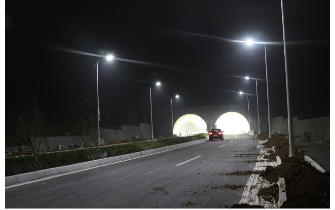
- for Road, China
